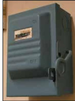
The easiest way to disconnect a studio kiln is with an electrical shutoff box. It should be installed near the kiln.
