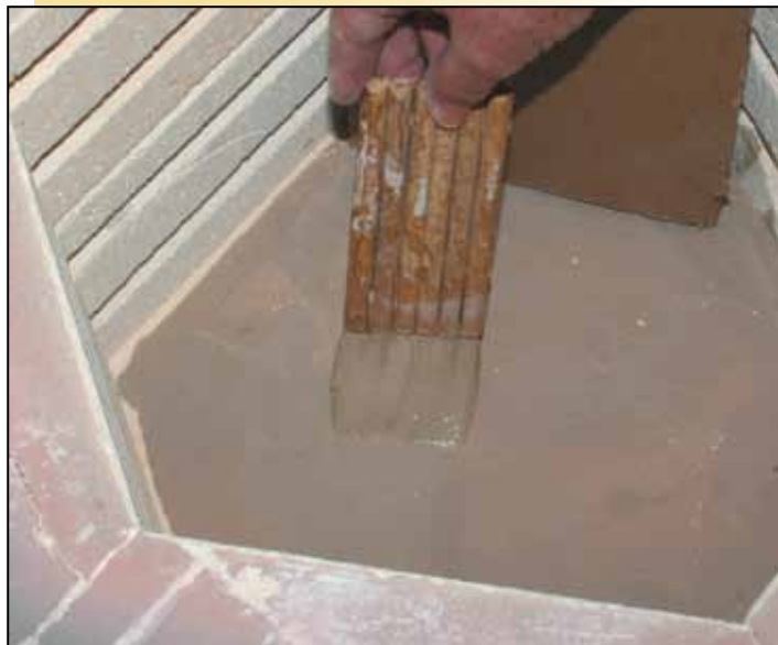
Avoid contaminating sidewall elements when coating the firebrick bottom. Photo courtesy of Paragon Industries, L.P.
